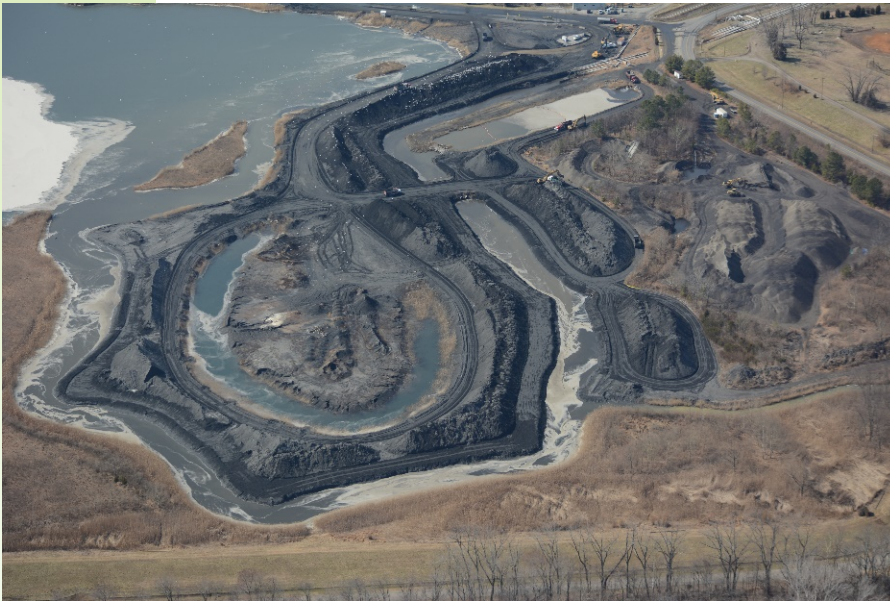
Coal ash storage at Dominion's Chesterfield Power Station facility, Virginia. Credit: James River Association.
