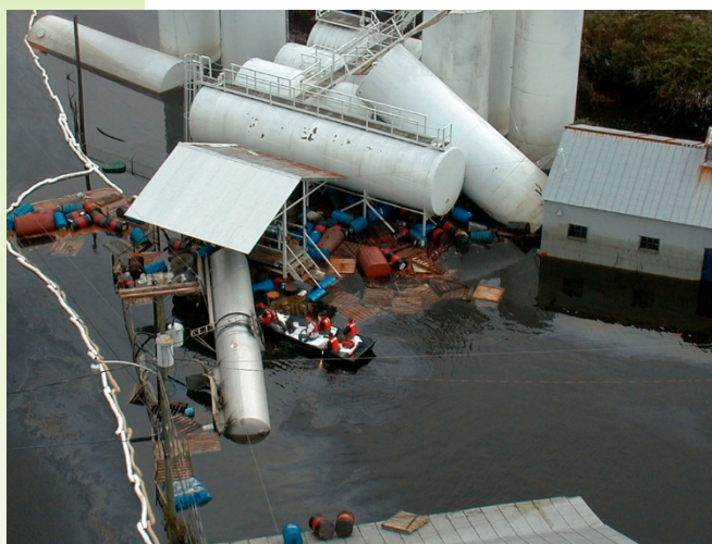
In 1999, flooding from Hurricane Floyd toppled storage tanks and carried away oil drums, resulting in floodwater contamination in Franklin, Virginia. Credit: Liz Roll/FEMA News Photo.
