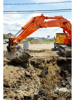
Sam, a backhoe operator, is working at the site to help dig a trench to lay pipes. While operating the backhoe, Sam misjudges the distance of power lines immediately overhead and makes contact with the live lines. Unaware of this, Carol, another worker at the site, attaches a chain to the bucket on the backhoe. When she makes contact with the backhoe, Carol is fatally
